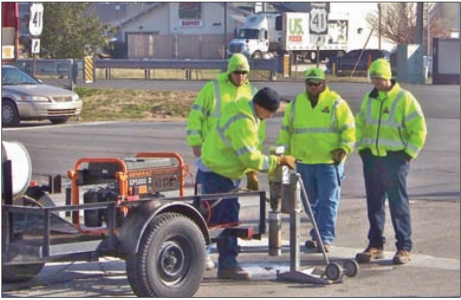
KENTUCKY TRANSPORTATION CABINET Above, workers with a Kentucky Transportation road crew install a new "puck" traffic-detection device at an intersection in Hopkinsville. At right, the device, which is buried in the pavement and covered with epoxy, is shown.
